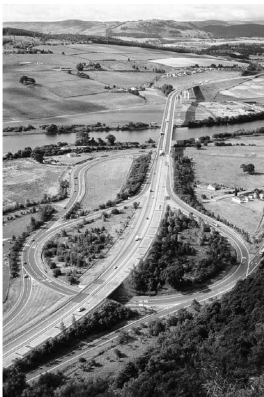
FIGURE 10 Motorway junction, Perth, Scotland
